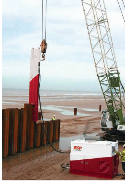
Above: Various SL30 Hammers fitted with legs and inserts for diving sheet piles. All are shown in crane suspended operation and powered by BSP Power Packs.
