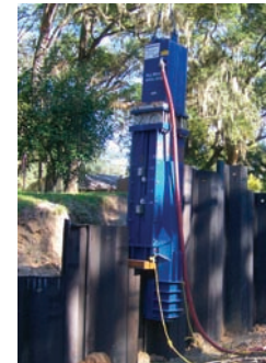
HAMMER WITH SHEET PILE SKIRTS
