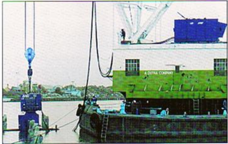
Model 450 Extracting 24" Concrete Pile
