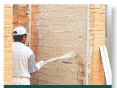
The versatile Quattro sprays mortars as well as pumps selfleveling underlayments.
