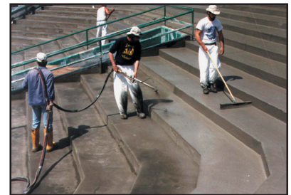
Concrete resurfacing.
