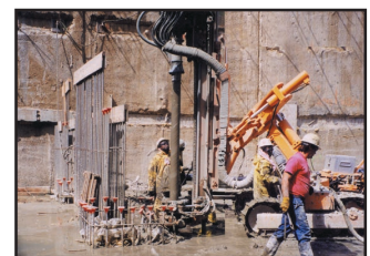
Fracturing/Regrouting
